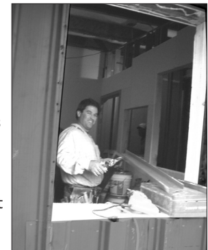
New windows with frames wrapped in metal siding to match the building.
