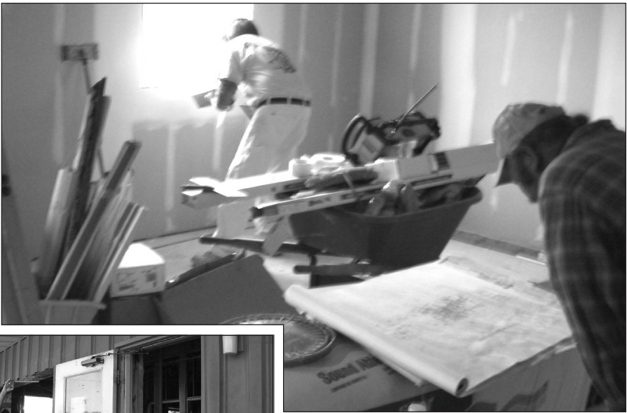
above: Finishing coats of sheet rock mud are applied, while blueprint specifications are given a final review. Power tools are picked up and organized. left: measurements are taken for new windows and doors.
