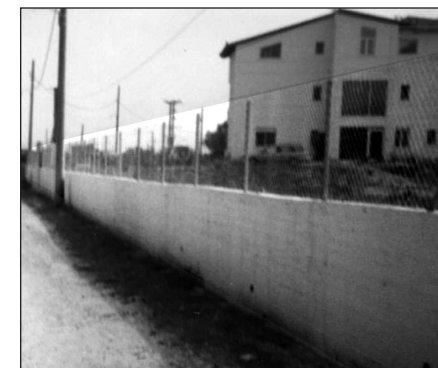
The mission team from Westpark Baptist reinforced the back wall with re-bar and added chain link fencing across the top of the front wall pictured above.
